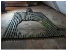
**T86 Roof Decking Laid Out after Removal** The cabin roof decking has been removed from the T86, leaving it in position would have posed a hazard.
